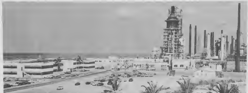
Refinery view before construction of the Hydrodesulfurization Complex.
